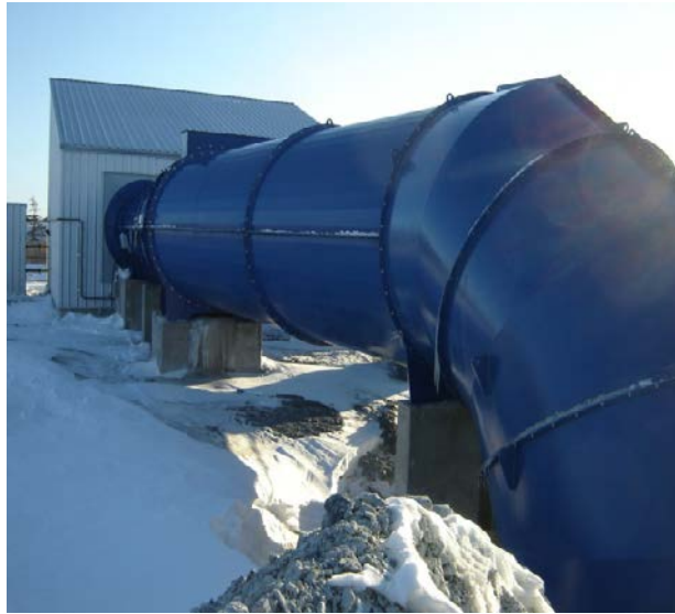
Figure 3 - New surface fresh air fan installation
