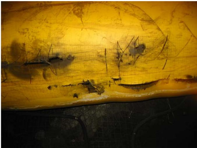
Figure 8. Severe leakage due to damage by equipment.
