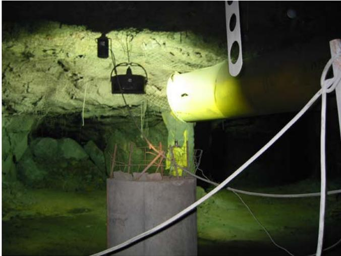
Figure 1. The end of the ventilation column should be kept as close to the face as possible.
