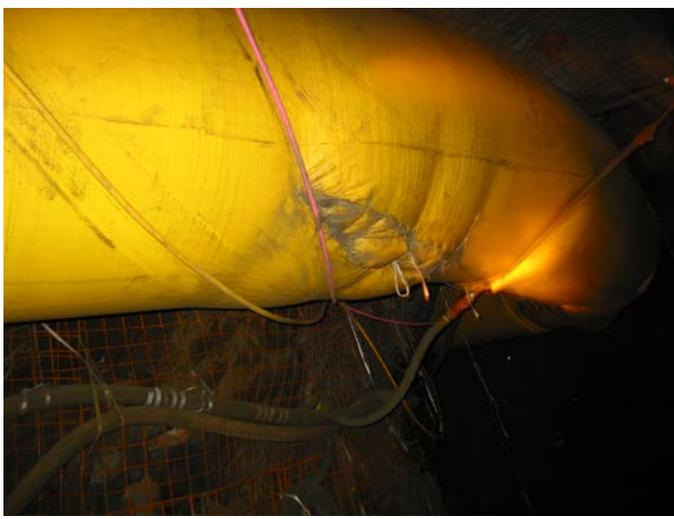
Figure 9. Stitching used to repair damage to tubing.
