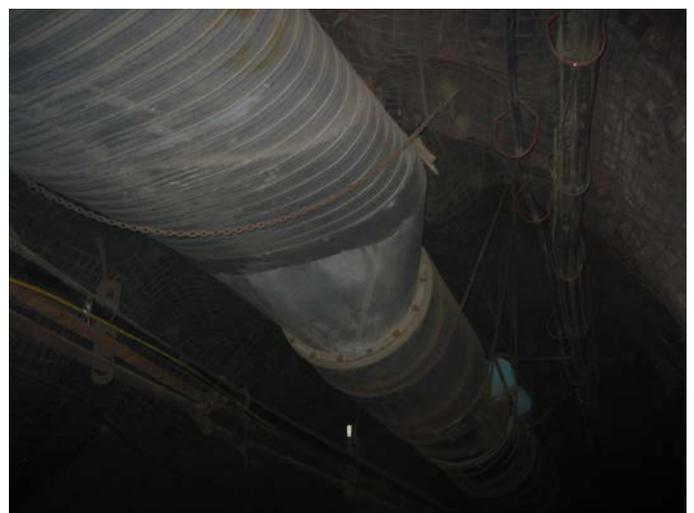
Figure 4. Circular and oval rigid duct in an exhaust system.
